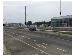
1 - LOOKING TOWARDS BOWEN ROAD
